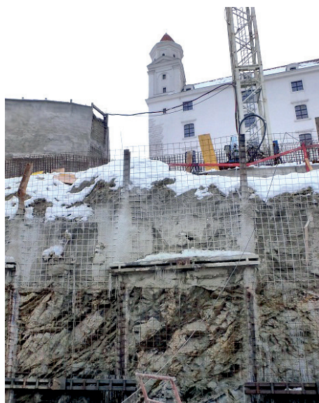
Fig. 1.6 The excavation works in the area of the Bratislava Castle testify to a multiphase neoid tectonic failures of the Castle Cliff; a) brittle deformation, prevailing failure directions dipping to the east; (b) young failure accompanied by the development of a light tectonic clay (scale – geological hammer)
