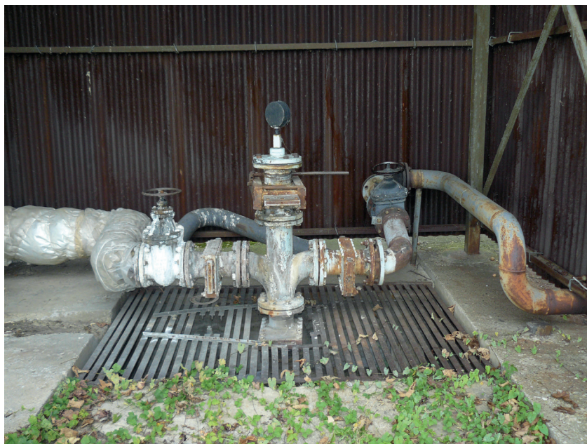
Fig. 5.2 Collar of one of the most valuable geothermal wells of the Central Depression of the Danube Basin – well FGT-1 in Topolníky (photo: D. Marcin, 2010)
